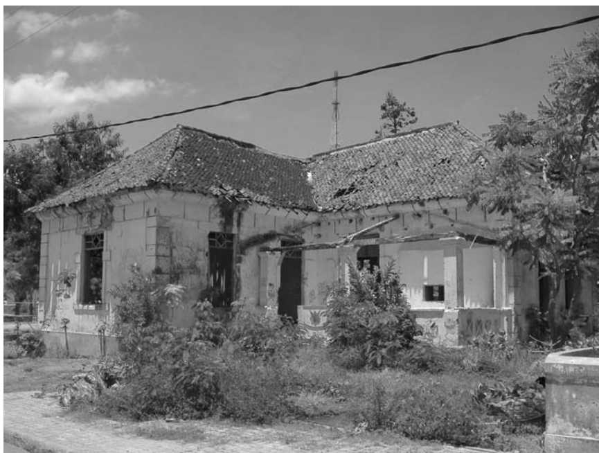
Figure 6.7 Destroyed buildings in Timor-Leste.
