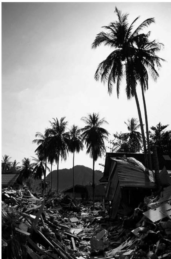
Figure 8.6 Tsunami damage on Khao Phi Phi, Thailand, January 2005.
