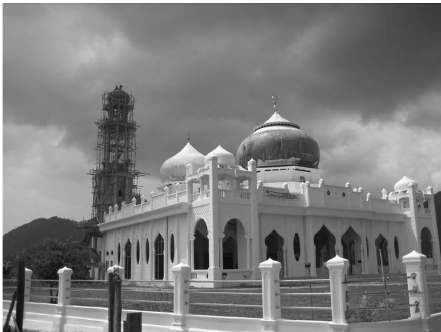
Figure 5.3 Rahmatullah Mosque, Lampuuk, Aceh, being rebuilt after 2004 tsunami.
