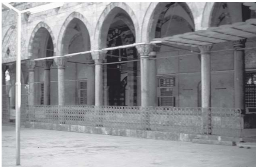
Pl. 15. 'Ādiliyya complex. Portico of the Mosque.
