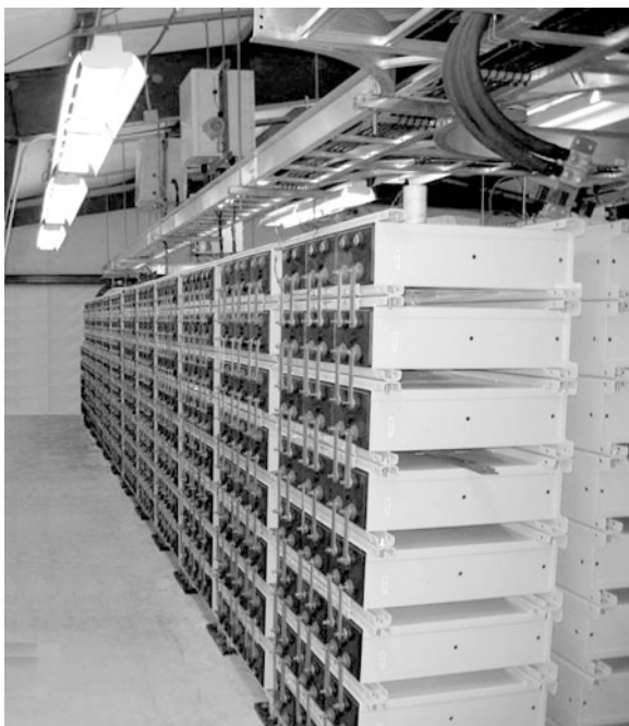
Fig. 9.3 A portion of the BESS at Metlakatla, Alaska that uses GNB ABSOLYTE IIP 100A75 modules. Seen is one bank of a back-to-back row
