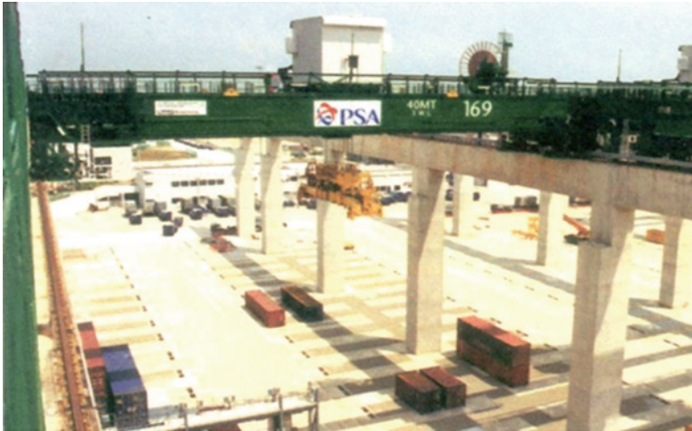
Fig. 18.3 Singapore's remote crane control system for freight/container handling in the yard
