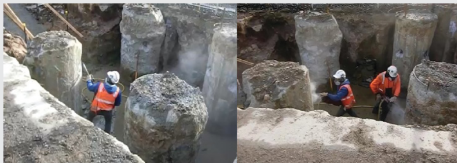
Figure 9.1 Using a hand-held pneumatic breaker to break down concrete pile heads.
