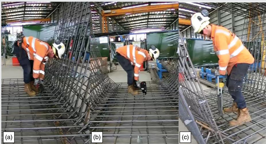
Figure 8.3 Steelfixing at ground level with (a) a conventional pincer-cutter tool, (b) a power-tying tool, and (c) a long-handled stapler tool.
