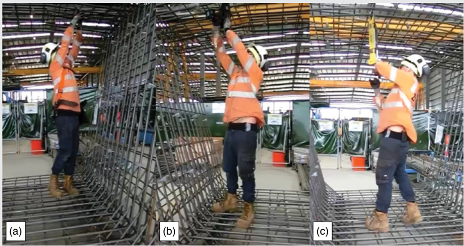
Figure 8.7 Steelfixing above shoulder height with (a) a conventional pincer-cutter tool, (b) a power-tying tool, and (c) a long-handled stapler tool.
