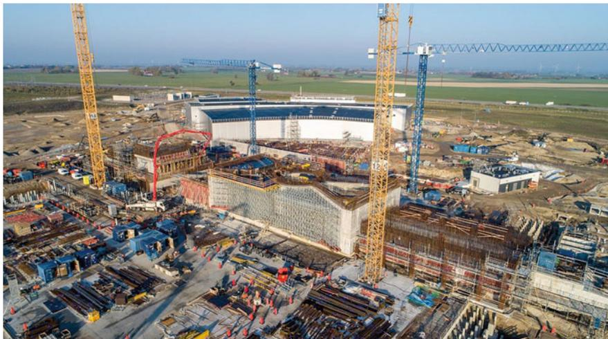
**Fig. 1** ESS under construction in Lund, Sweden. The central concrete structure will house the neutron production target
