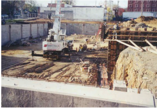
Fig. 3-11. Basement Wall under Construction, SCMB
