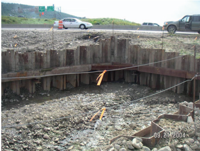
Fig. 5-11. Sheet Pile Cell
