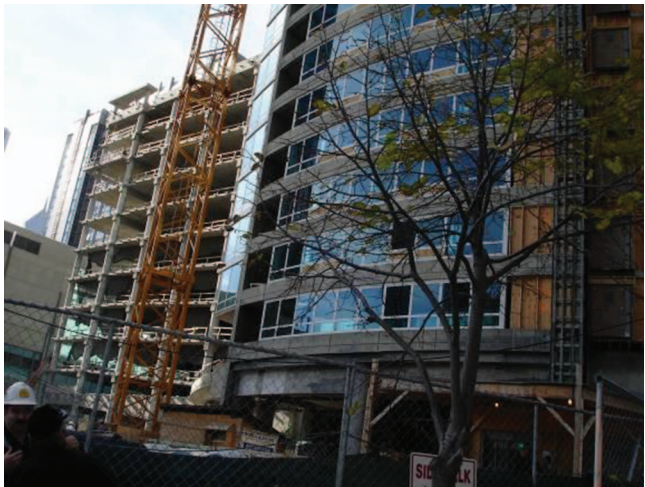
Fig. 8-7. Sealing and Enclosing a Building with Permanent Windows
