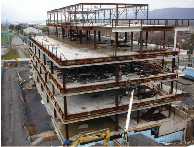
Fig. 6-10. Use of the Third Floor as a Semipermanent Storage Area
