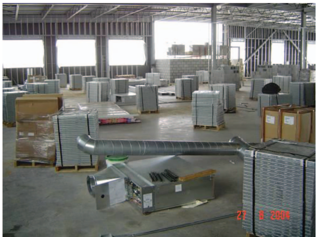
Fig. 6-6. Ineffective Application of Preloading
