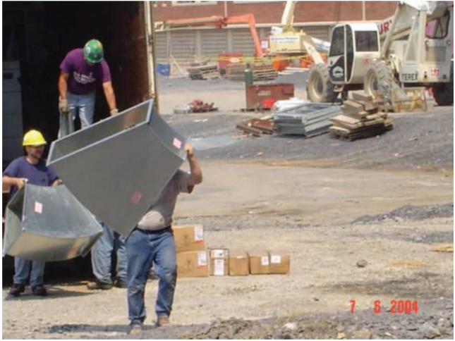
Fig. 6-19. Carrying Duct One Piece at a Time
