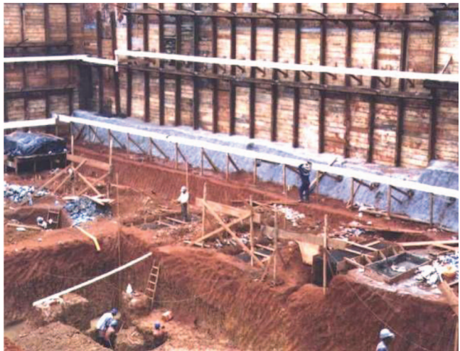
Fig. 5-6. Drainage of Facility Footprint
