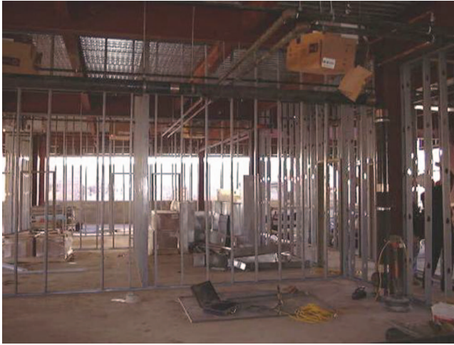
Fig. 9-3. Partition Walls Installed before Ceiling Work Is Complete
