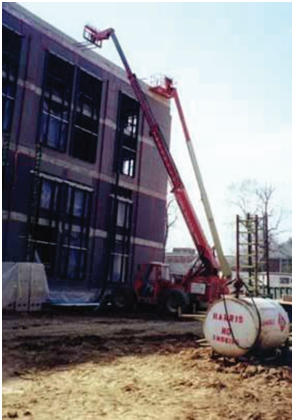
Fig. 6-25. Use of a High Lift to Move Materials into the Building, Paterno Library, Pennsylvania State University, State College, PA
