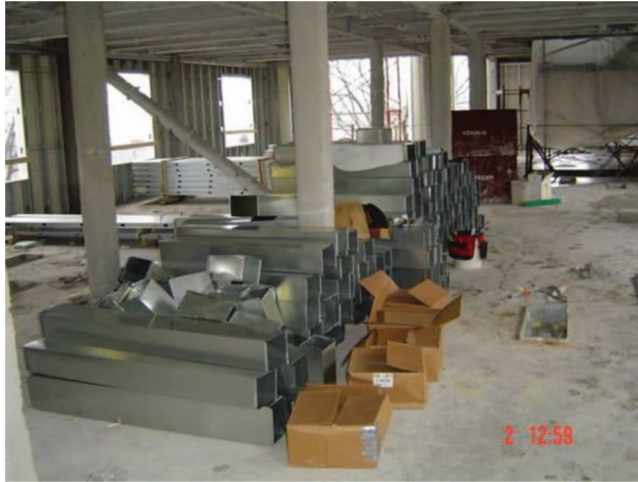
Fig. 6-8. Use of Constructed Areas for Storage
