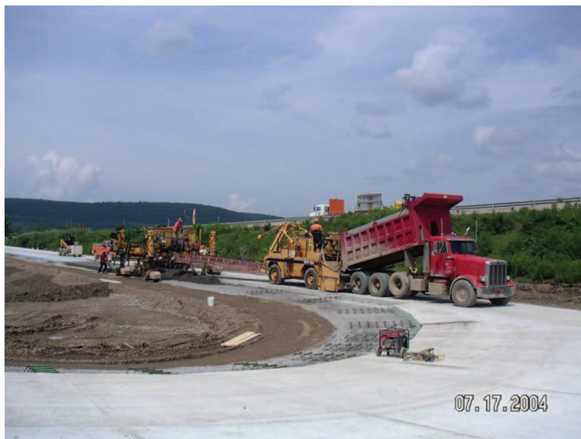
Fig. 5-17. Concrete Paving Operation
