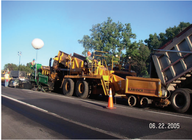
Fig. 5-18. Asphalt Paving Operation
