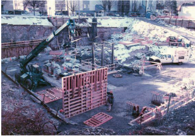
Fig. 7-24. Erection of Gang Forms Using 30-Ton Crane
