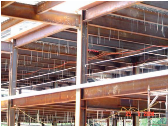
Fig. 7-4. Workers Have Done Hanger Erection Only this Day, Smeal College of Business, State College, Pennsylvania
