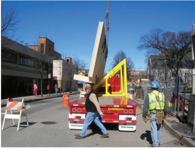
Fig. 6-23. Erecting Precast Element Directly from the Truck (Right Piece, Right Time)
