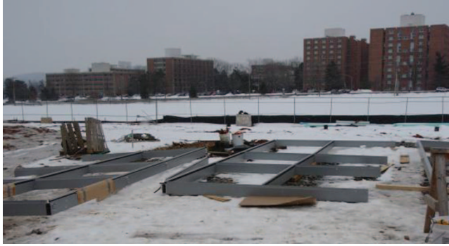
Fig. 7-12. Support Frame Subassembly for Curtain Wall, Dickinson Law School, Carlisle, Pennsylvania
