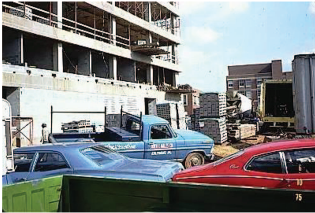
Fig. 6-12. Congested Staging Area, State College, PA
