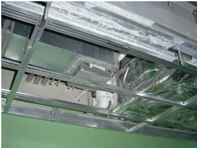
Fig. 9-1. Ceiling Grid Installed before Piping and Conduit Work
