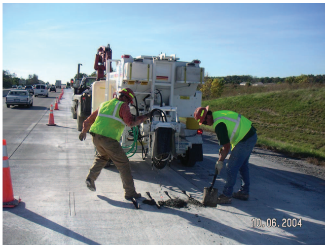
Fig. 5-16. Dowel Bar Retrofit, Concrete Pavement Repair
