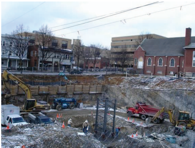
Fig. 7-25. Tower Crane Being Erected Beneath a Power Line
