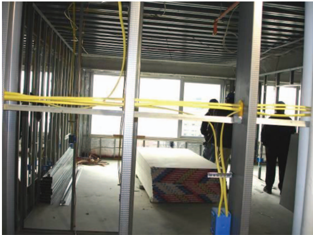
Fig. 7-15. Good Drywall Erection Practices Showing Uncluttered Work Face
