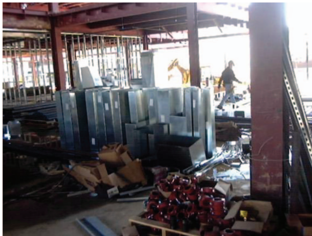
Fig. 6-9. Storage of Materials in the Building Interior, SCMB
