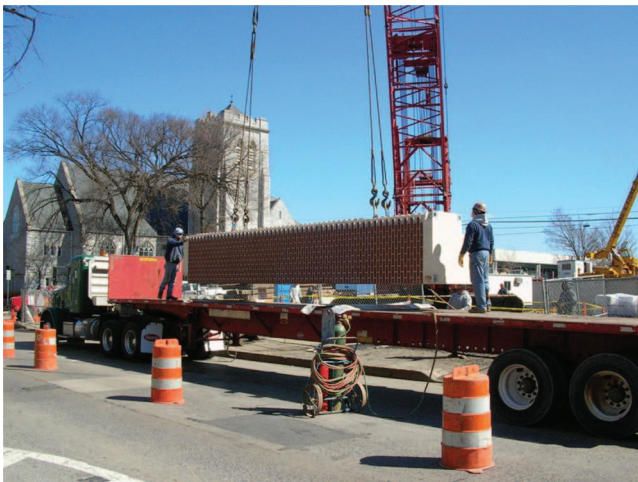
Fig. 6-11. Erection of a Precast Column Directly from the Delivery Truck
