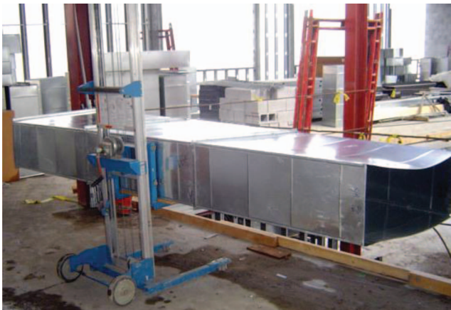
Fig. 2-2. Three-Piece Subassembly of Duct, Redifer Commons, State College, PA
