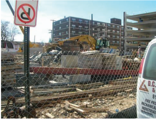
Fig. 4-4. Actual Site Conditions, Phase 2, Beaver Avenue Parking Garage
