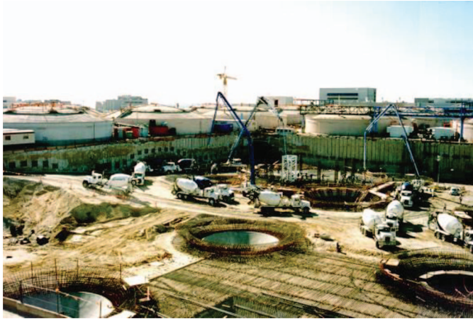
Fig. 12-5. Construction of Cones and Mat Slab for Batteries D1 and D2
