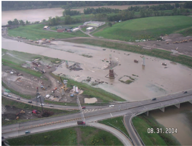
Fig. 5-15. The Effect of Flooding on a Construction Project
