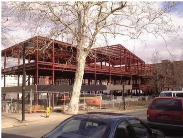
Fig. 3-2. State College Municipal Building (SCMB) during Construction
