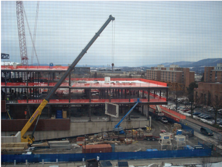
Fig. 3-26. Panel Erection Showing Congested Work Area, Millennium Science Complex
