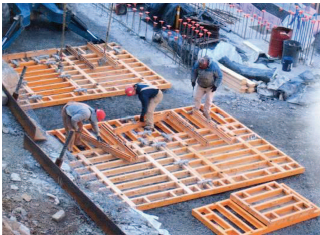
Fig. 7-23. Assembly of Gang Forms
