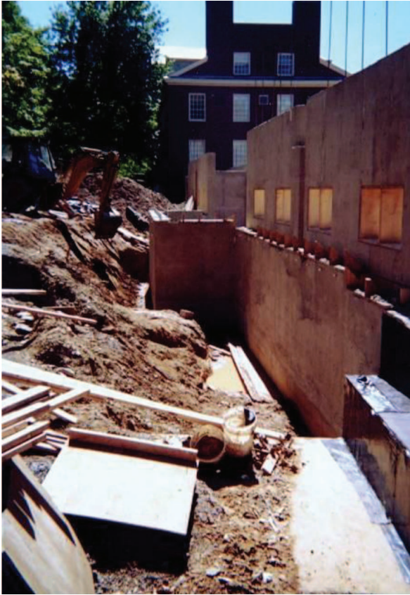
Fig. 6-16. Late Backfilling, O'Leary, Lewisburg, PA
