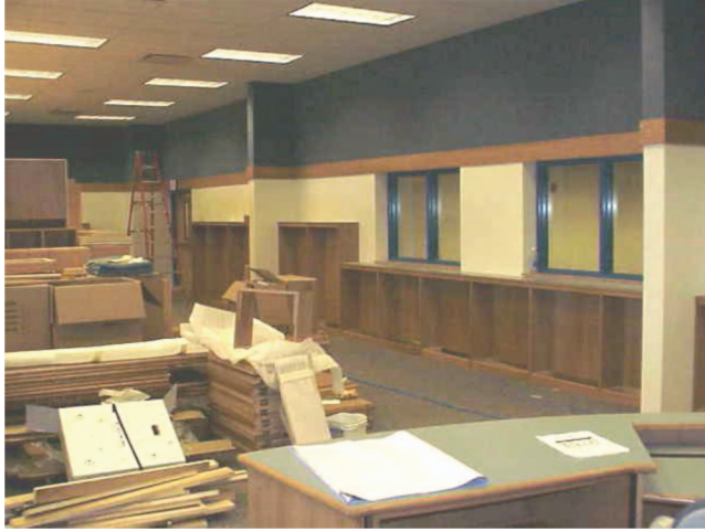
Fig. 6-17. Library Storage, West Point School Renovation, Pittsburgh, PA
