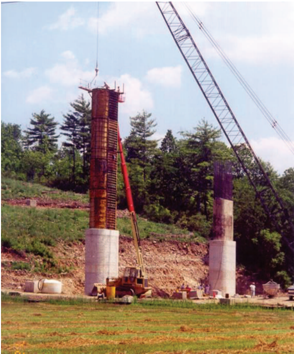
Fig. 7-21. Piers, Logan Branch Bridge, Central Pennsylvania
