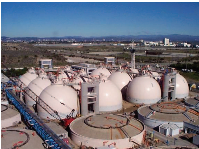
Fig. 12-4. Hyperion Site under Construction, Batteries D1 and D2
