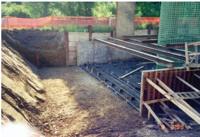
Fig. 7-19. Footers, Logan Branch Bridge, Bellefonte, PA
