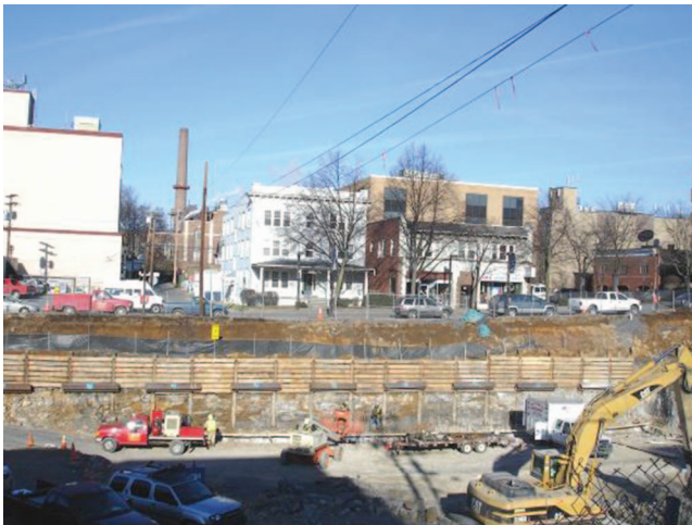
Fig. 8-5. Aboveground Power Line that Has Not Been Relocated
