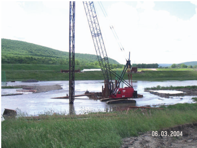
Fig. 5-14. Pile Driving in Flooded Conditions
