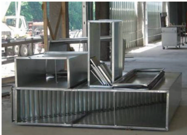
Fig. 6-5. Preloading of Duct
