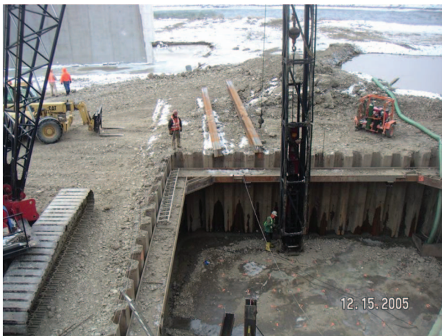
Fig. 5-12. H-Pile Driving
