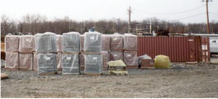
Fig. 5-10. Proper Storage Practices to Protect Materials from the Weather
