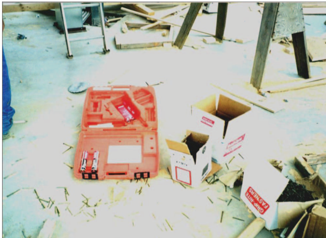
Fig. 11-3. Sloppy Housekeeping at the Work Face
