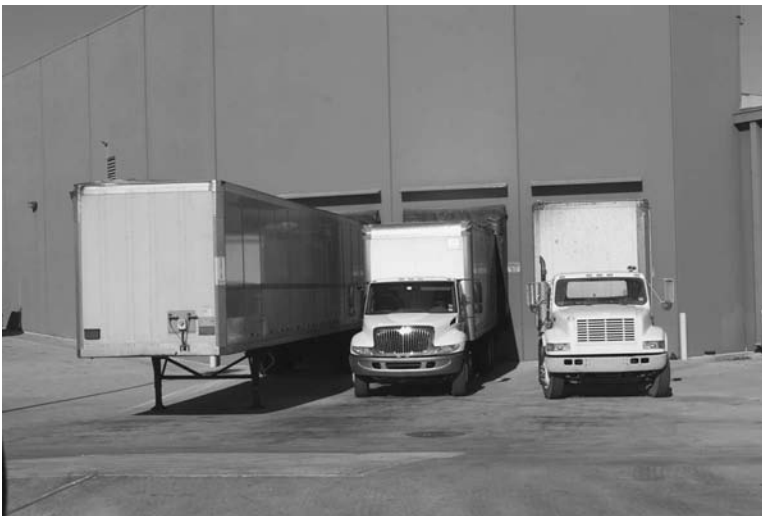
Figure 11.1 Security loading docks are commonly used as employee and vendor exits and entrances—they can also be opportunities for theft.
