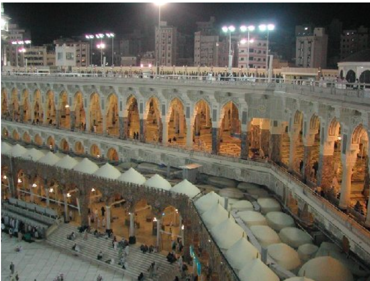
Fig. 5. Example image depicting the complex structures of the al-Haram Mosque
