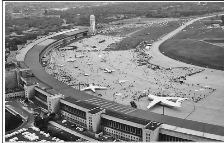
Figure 15: Inverted curvilinear terminal with open apron at Berlin-Tempelhof airport (Lopez, 1984)
