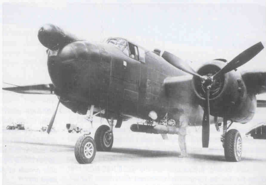
Above: These PBJ-1Js are painted in the tri-color camouflage scheme and have radomes on their starboard wing tips. They also have the bombardier's nose which was standard on most PBJ-1Js. (USAFM)
